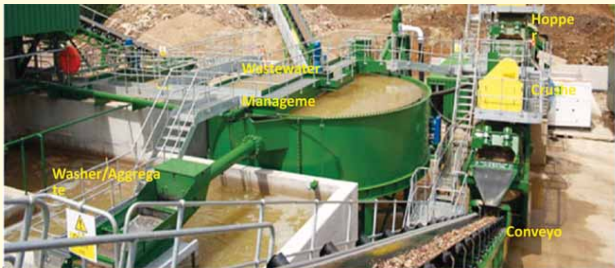
Figure 6.4.1 - C&D Waste recycling plant in Delhi
